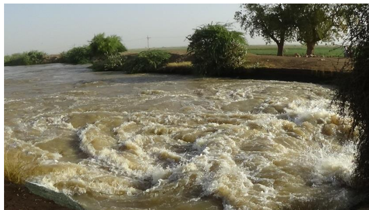
Photo 5: Bank erosion downstream large cross structures, February 2016
