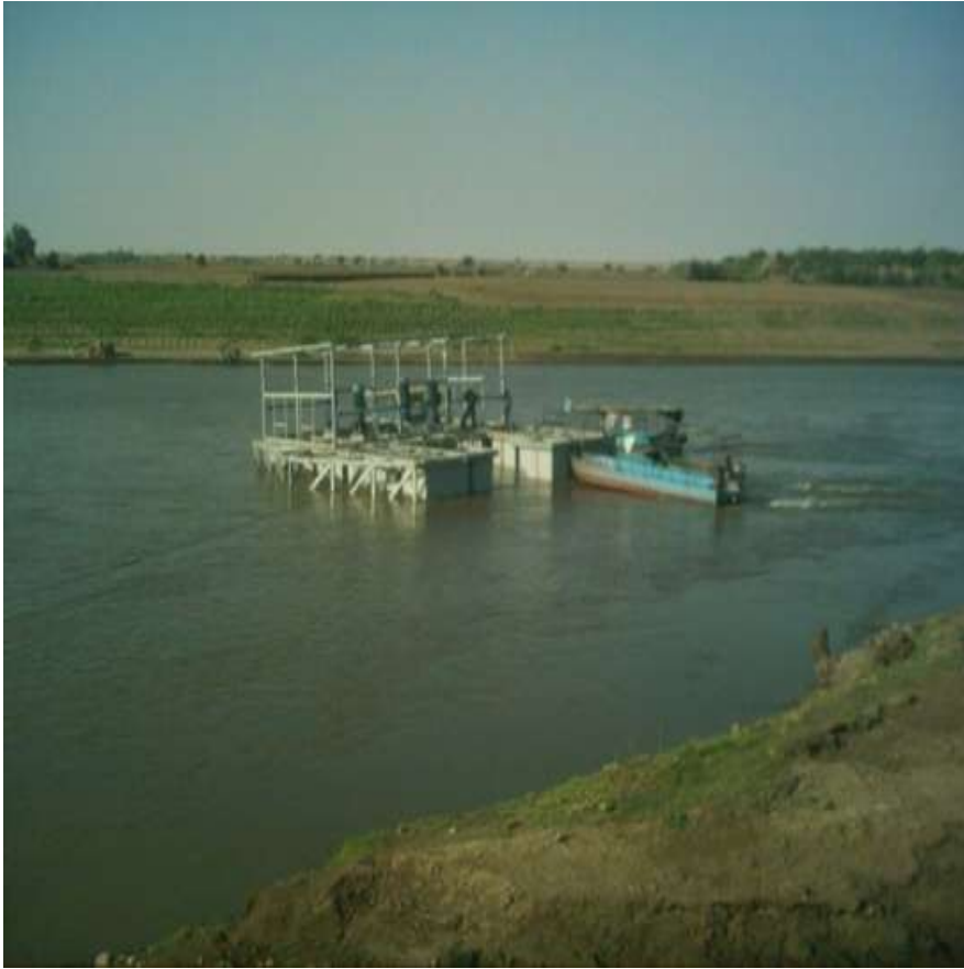
Pumping site location (2009)
