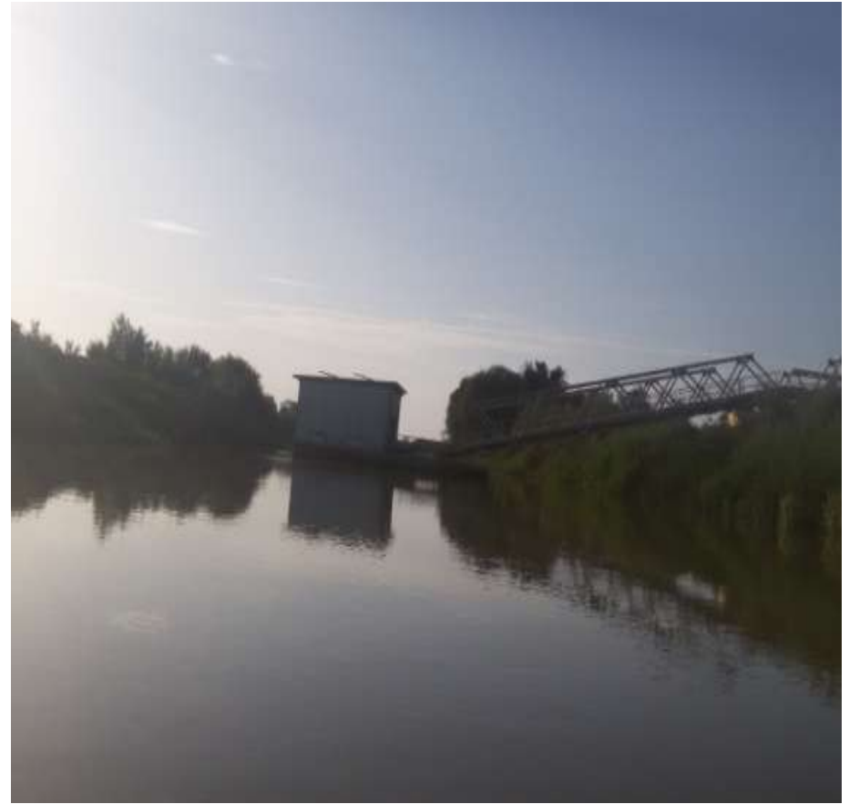
Pumping site location (2016)
