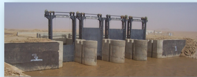
ROLLER SLUICE-GATES [RSG]
